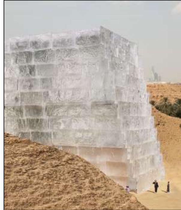
A Borosilicate Cast Glass Museum Facade in the Middle East | Agnes Koltay, Koltay Facades
